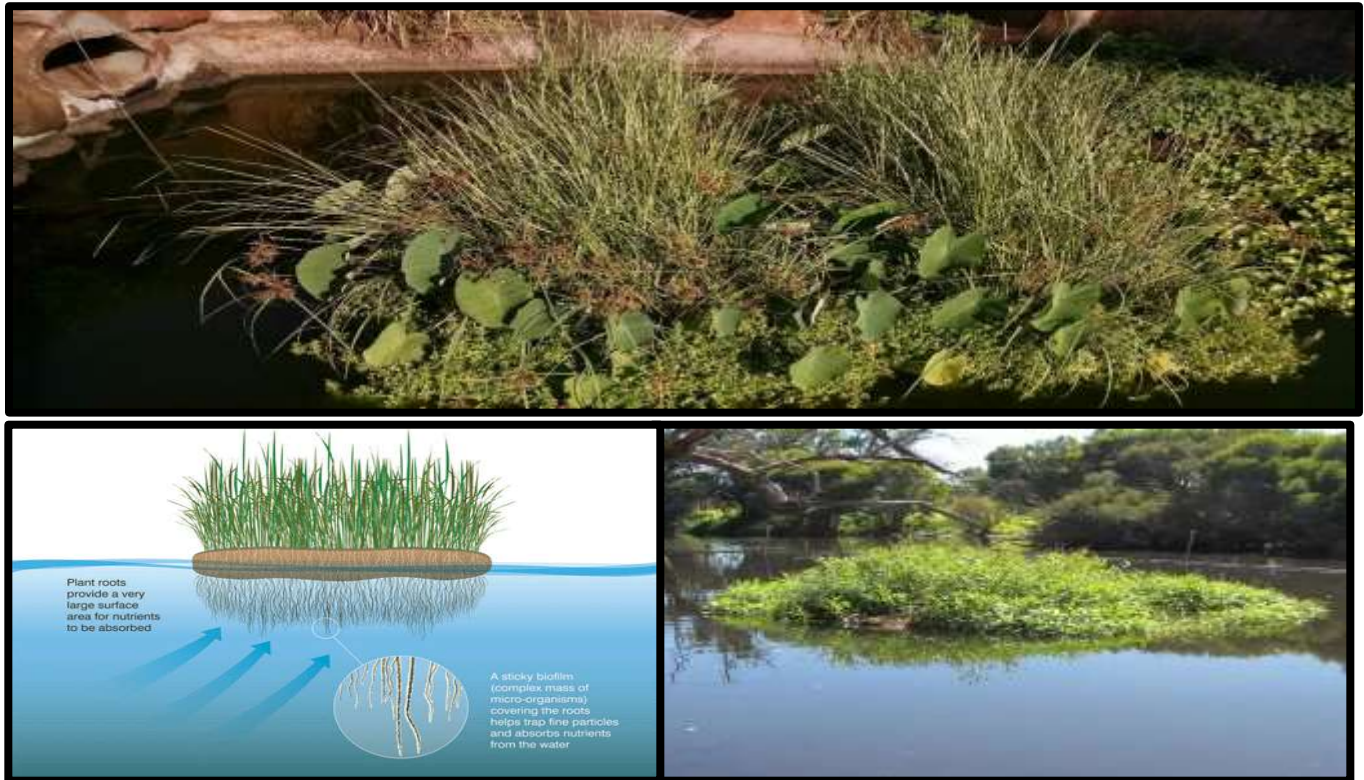
Figure 41. Floating Treatment Wetland
