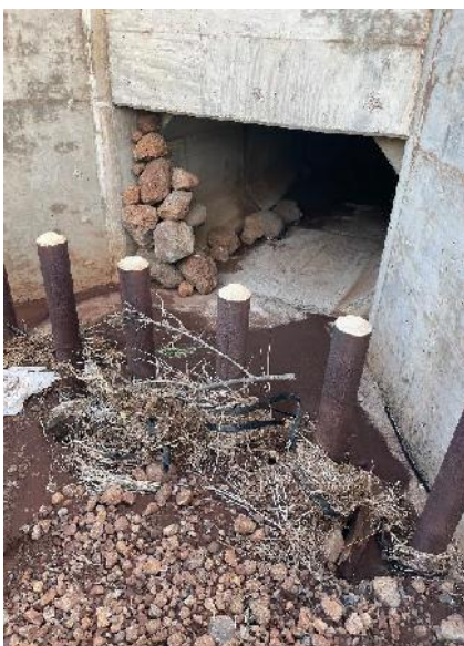
Wreck lines and sediment deposits at culvert entrance
