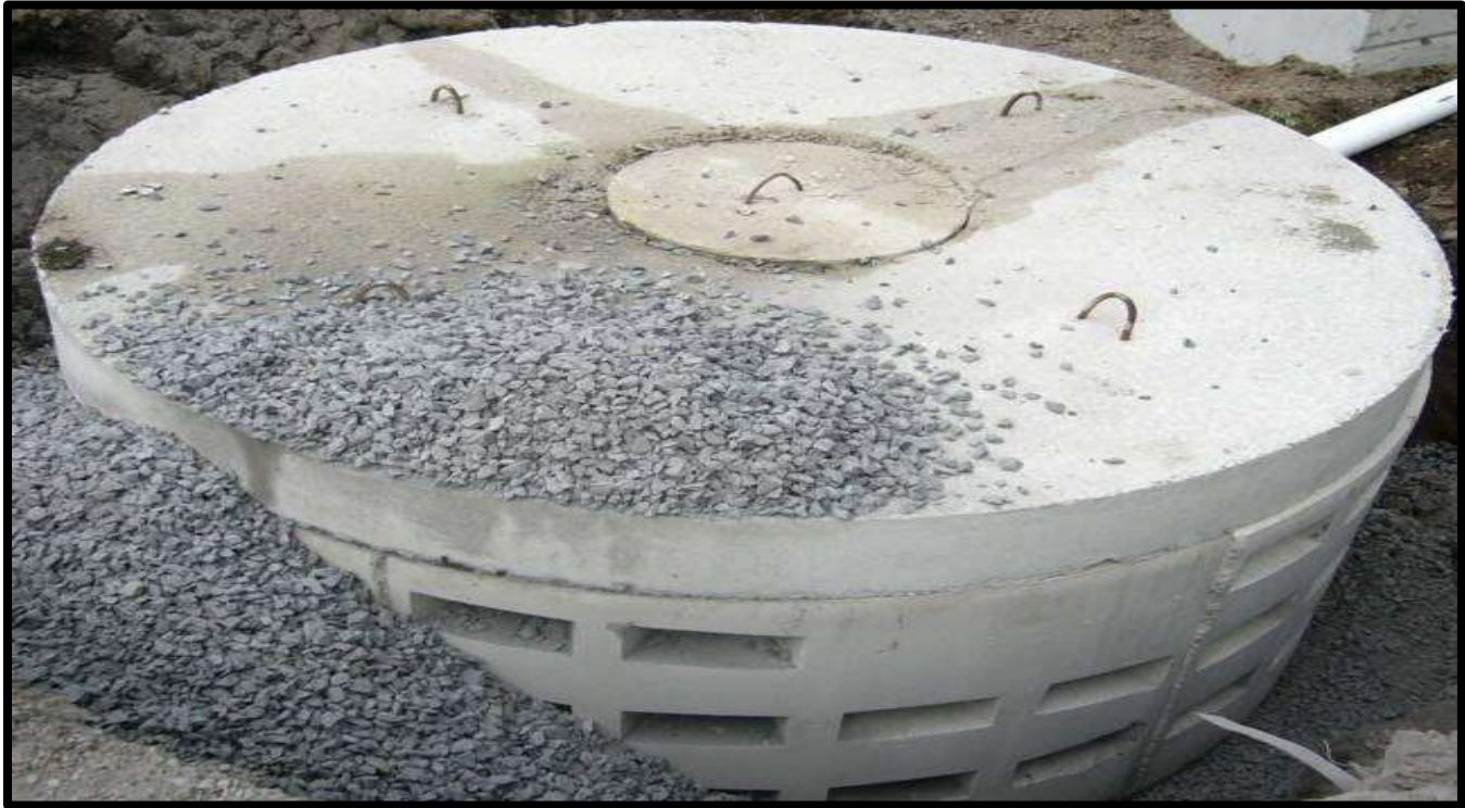
Figure 43. Stormwater Infiltration Well
