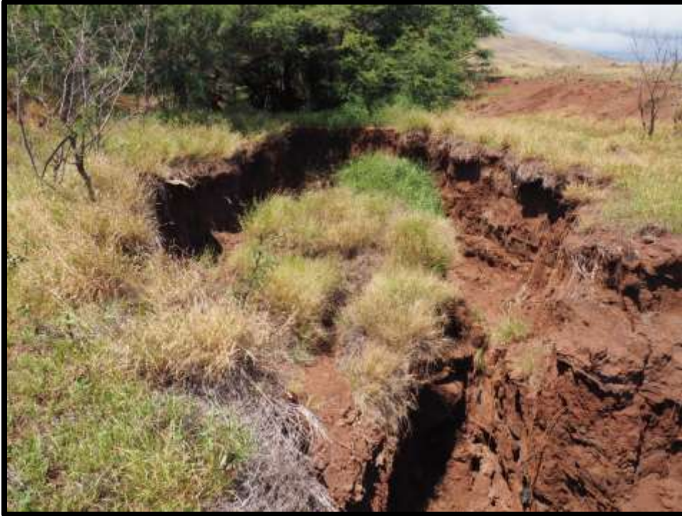
Figure 46. Current Mā‘alaea Gulch Head Cut Monitoring Station – March 2021
