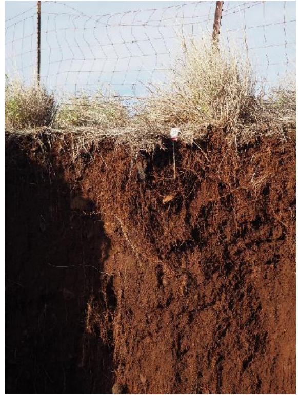
Exposed soil pin at array #9
