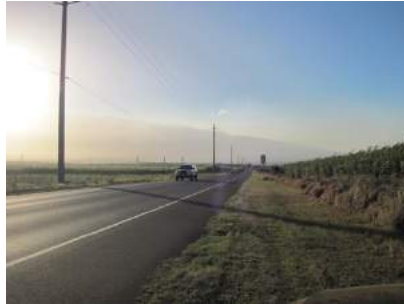
Highway 310 near Park and Ride, mowed shoulder on one side
