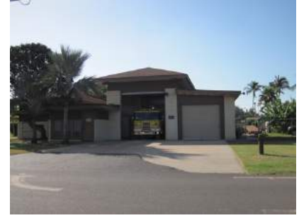
Kihei Fire Station
