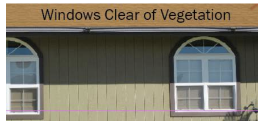
Figure 7. Keep windows free of vegetation to reduce likelihood of heat-caused breakage that lets embers into your home.
