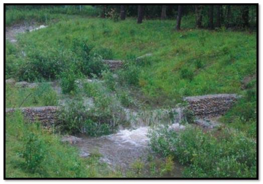
The following map provides an example for potential locations for gabion placement in Waiakoa Gulch (Figure 66. Waiakoa Gabions). Actual placement should be determined by topography, access for installation and maintenance, land ownership, and other factors. The life expectancy of gabion is based on the type of wire used to create the cage and not on the material used as filling. Typically, these cages are constructed of galvanized steel wire with a life expectancy of 50 years.
